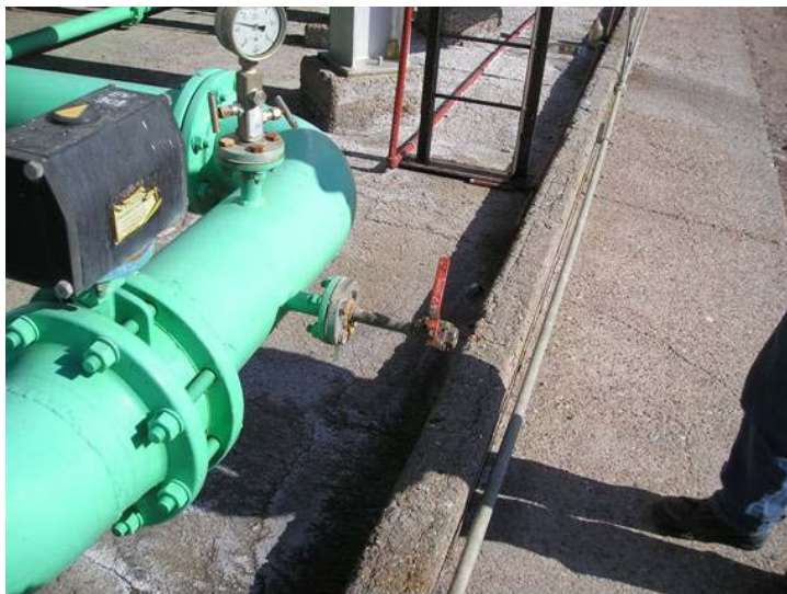
Figure 2-Valves show corrosion problems
